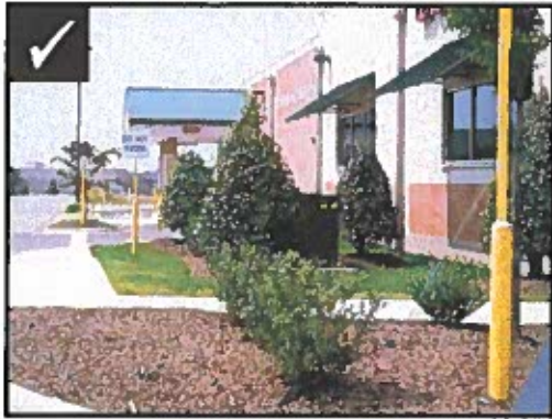
Mechanical Equipment Screened with Landscaping
