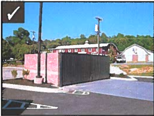
Solid Masonry Screen with Gates
