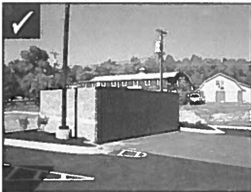
Solid Masonry Screen with Gates
