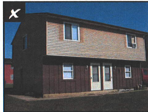
Entrance on Same Plane of Facade
