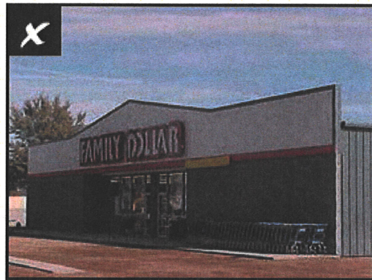
Standard Concrete Block and Metal Facades
