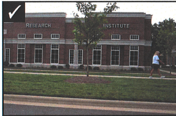
Parapet with Decorative Cap & Varied Roof Line
