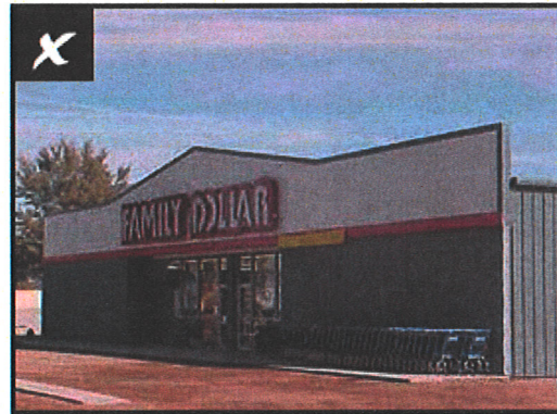
Parapet on Front Facade Only: No Decorative Cap
