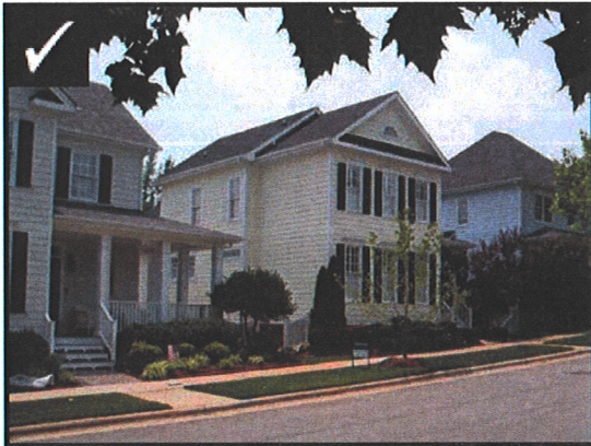
Approximately 12-inch Overhang
