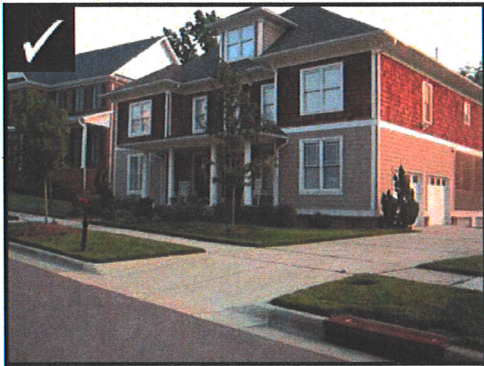
Wood Shingles and Clapboard Siding
