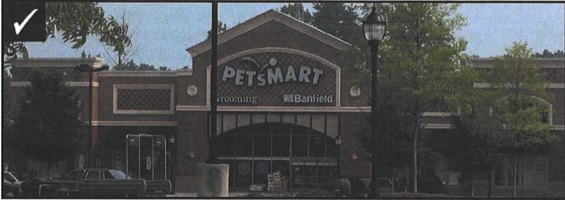
Facade with Recesses & Projections
